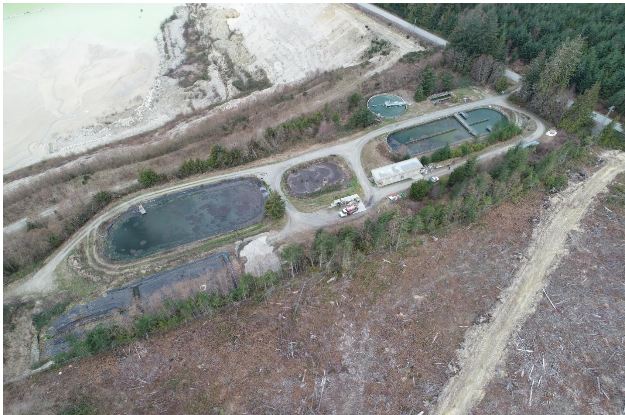
Figure 1: Dusty Road Septage Facility, facing northwest
