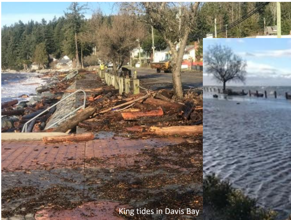
Flooding near Heritage Road and Fairway
