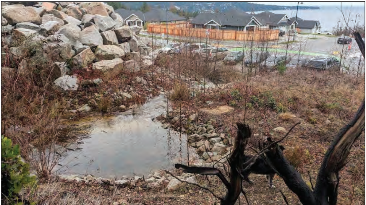
Photo 6. Stormwater management pond on Watercourse-1, at the north side of Derby Road upstream of the pipe.
