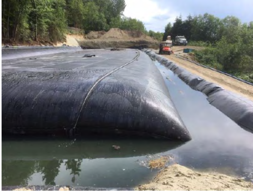
Photo 8-3 Geotubes at the Dusty Road Facility
